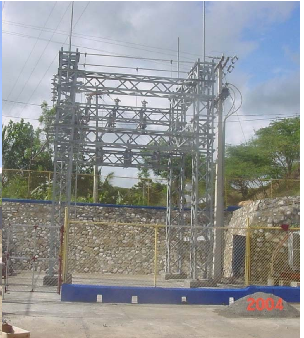
Two of the Dominican Republic 12.5 KV lattice structures after field installation were completed.
