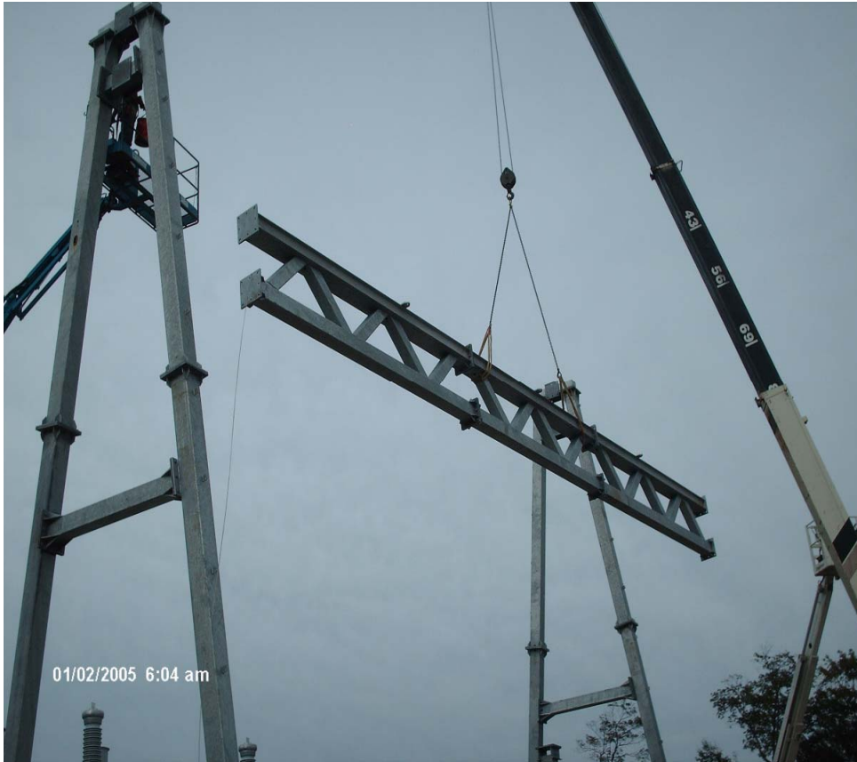
Erecting the beam of the 230 KV A-Frame deadend at Prince Windfarm Phase 2.
