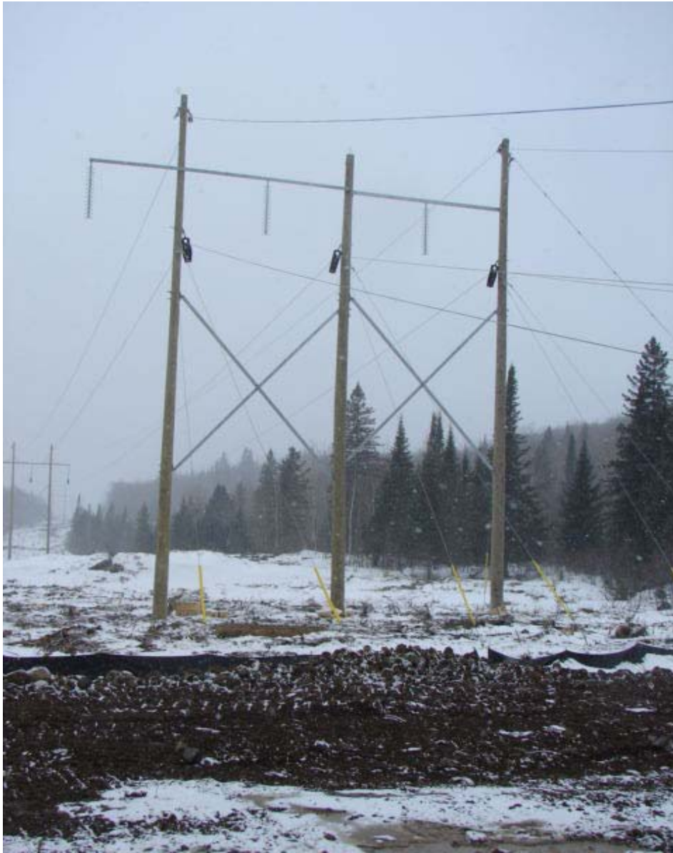
230 KV transmission line steel cross arms and cross braces for angle and tangent structures leading to Prince Windfarm.
