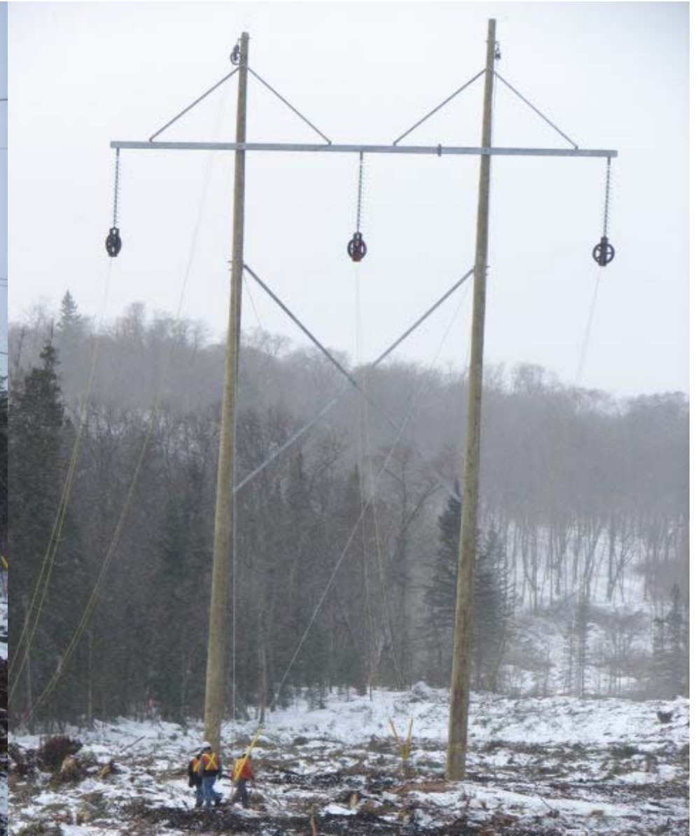
230 KV transmission line steel cross arms and cross braces for angle and tangent structures leading to Prince Windfarm.
