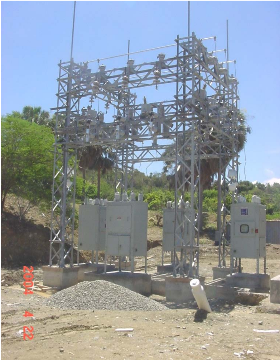
Two of the Dominican Republic 12.5 KV lattice structures after field installation were completed.
