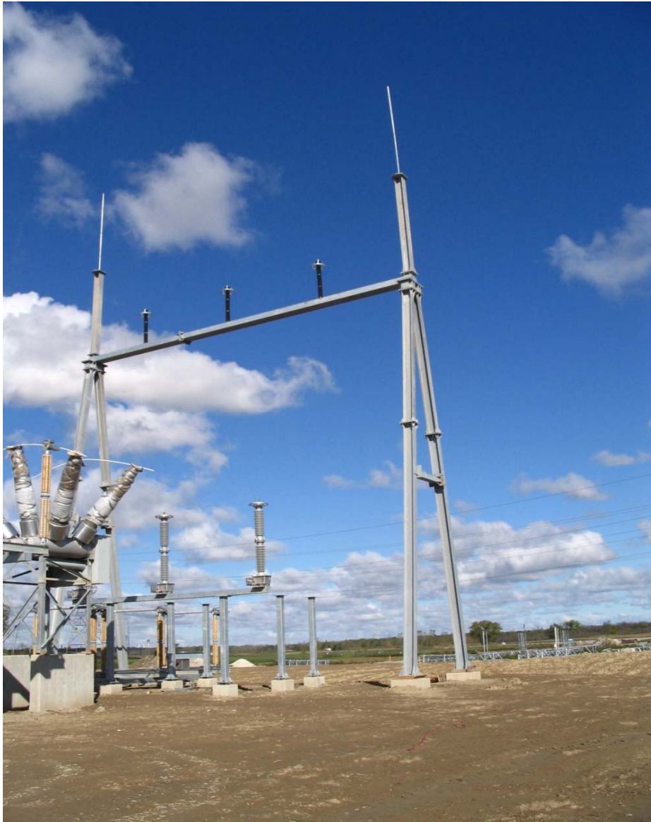
230 KV deadend structure using I beam columns for high loading condition.
