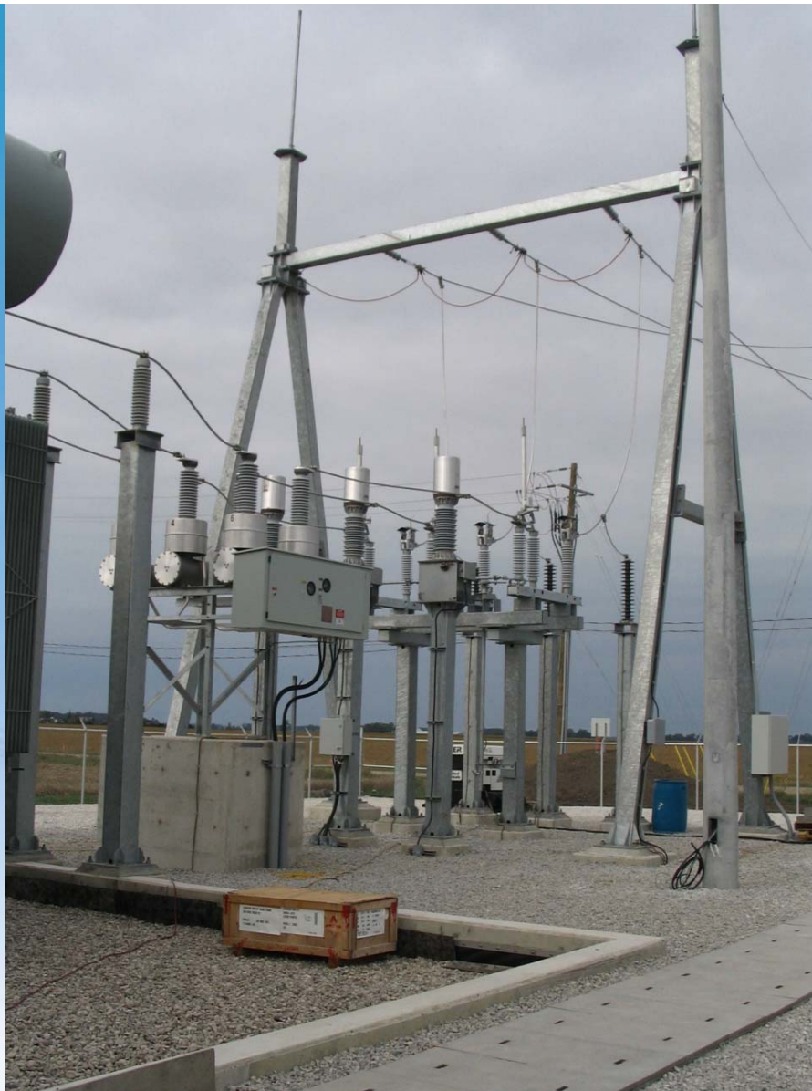
69 KV disconnect switch, metering stands and A-Frame deadend structure.
