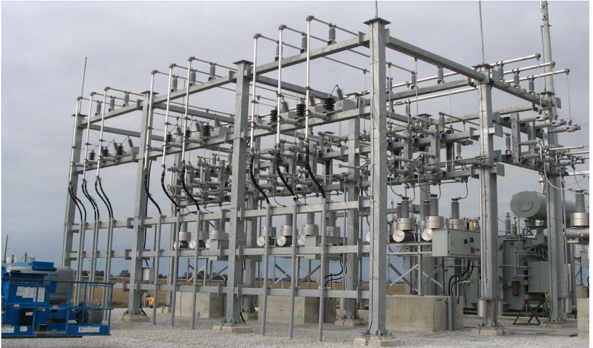
Riply windfarm 34.5 KV 6-bay structure collecting power from 39 turbines to feed the 69 KV transformer.
