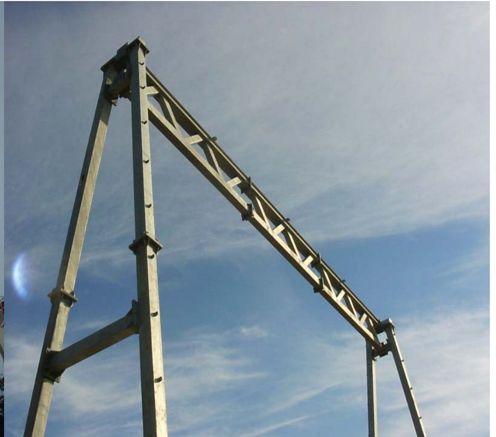
Erecting the beam of the 230 KV A-Frame deadend at Prince Windfarm Phase 2.
