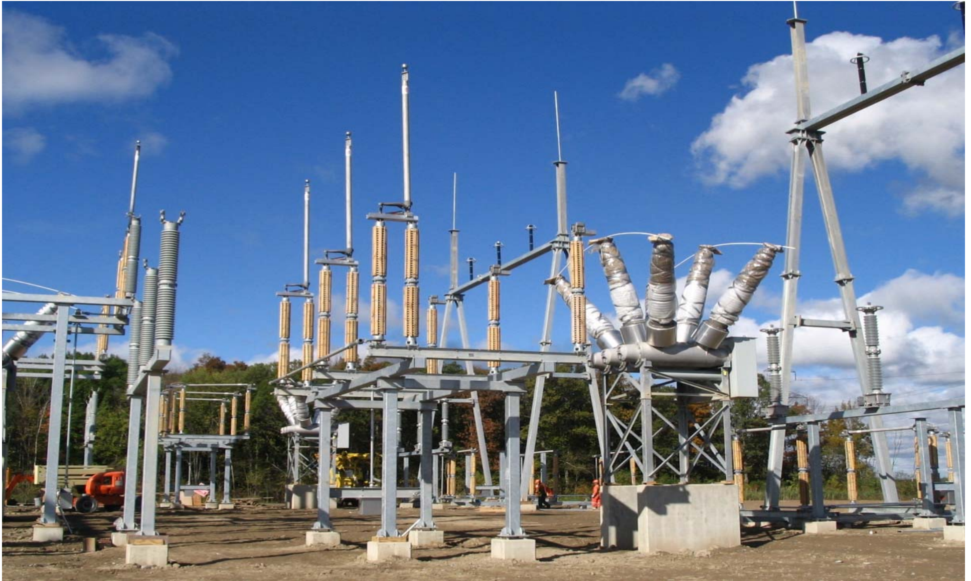
Partial view of the switchyard at St. Clair site showing 230 KV disconnect switches, circuit breakers and A-frame deadend structures in the background.
